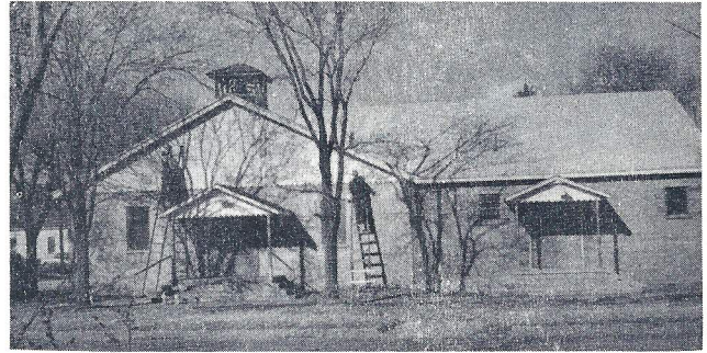
THE CHAPEL in Guthrie gets some paint before the assembly meeting.
